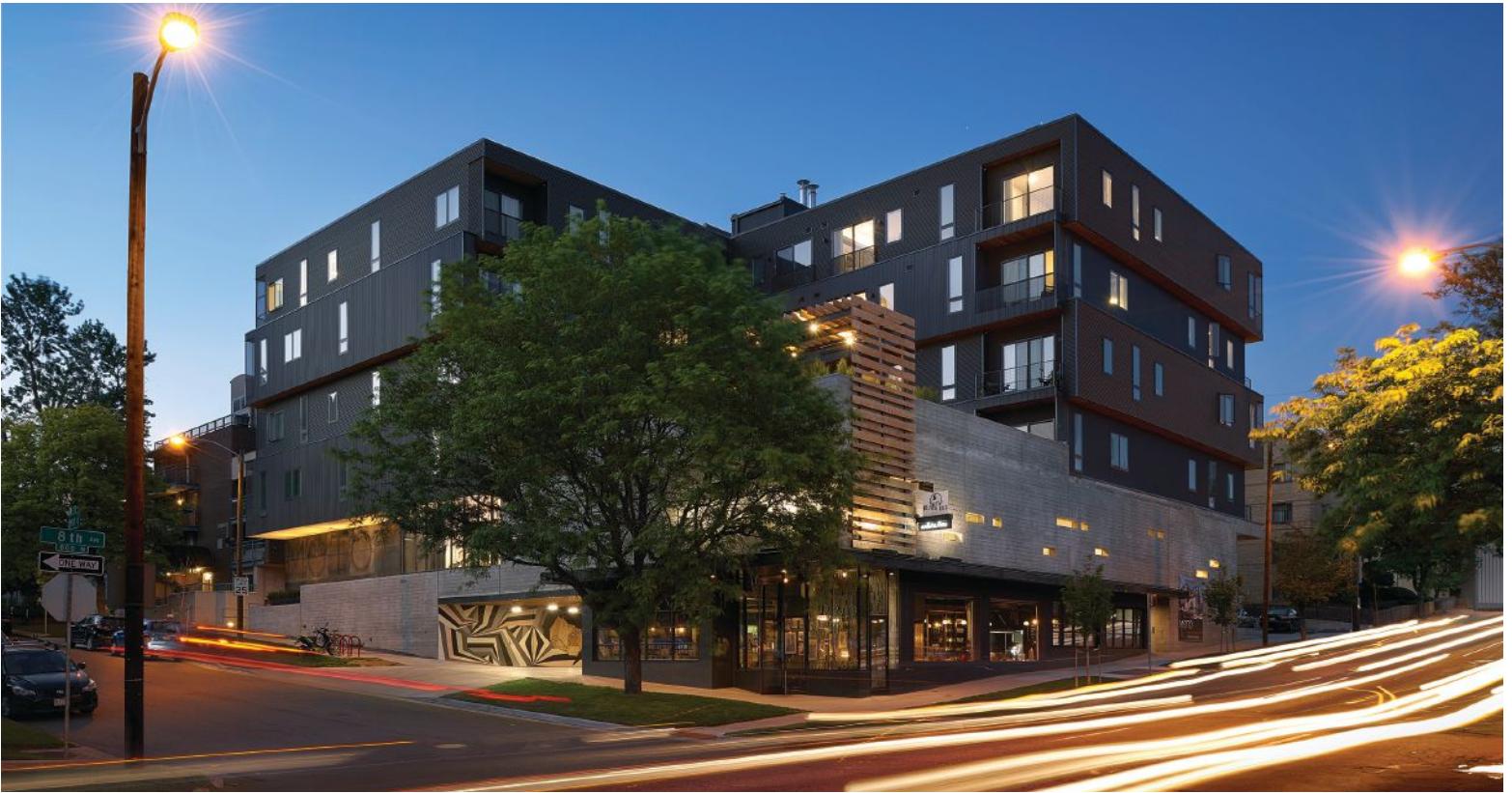
At MOTO, a panelized light frame wood wall system allowed each level to be framed in about a week and the entire project in less than a month. Photo: Ryan Gobuty
