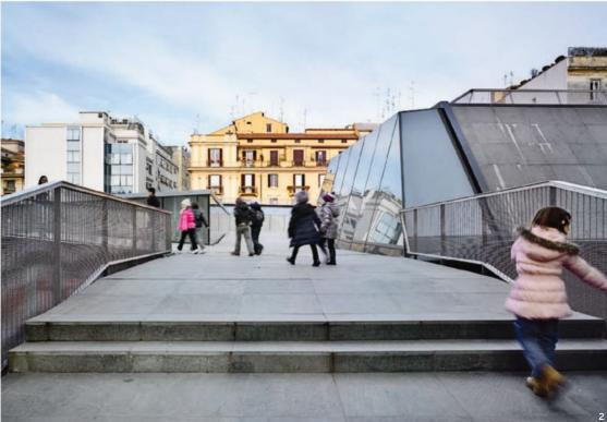
1 and 2. The architects created an artificial landscape on the museum's roof, placing a piazza there to connect the building to its historic context. The large skylight in the center of the piazza was designed to serve as a fountain with a sheet of water sliding over its surface, but it does not always work.
