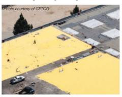
This thermoplastic roofing membrane was chosen as the best solution for cost and time saving for the roof renovation of the City of LA Police Department.
