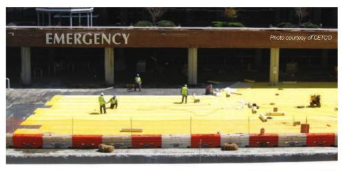
Workers installing thermoplastic membrane waterproofing system over the existing failed rubberized asphalt membrane on the split-slab deck of this hospital.
