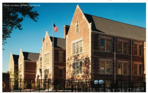
Window replacement for the William C. McGinnis Middle School in Perth Amboy, New Jersey, used operable aluminum clad wood double-hung windows with high-performance low-E glass. These windows also included a between-the-glass window blind treatment as a method to enhance daylight and reduce allergens in classrooms.
