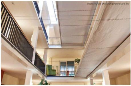
Shown here, typical fire- and smoke-rated flexible curtains partially closing in a horizontal application. Firerated curtains rated up to 2 hours can be constructed of stainless steel strengthened glass filament fabric.
