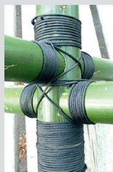
Traditional Joinery details – bamboo pinning, tying bamboos
