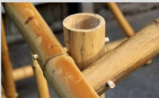
Traditional Joinery details – bamboo pinning, tying bamboos
