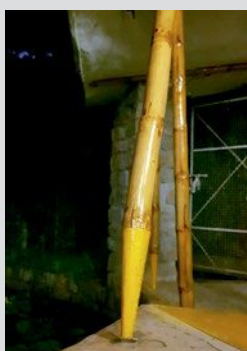
Depiction of boot (footing) and hat (roof projection) for bamboo
