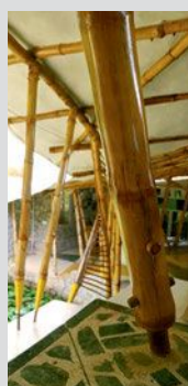
Finish of bamboo and showing fixing details
