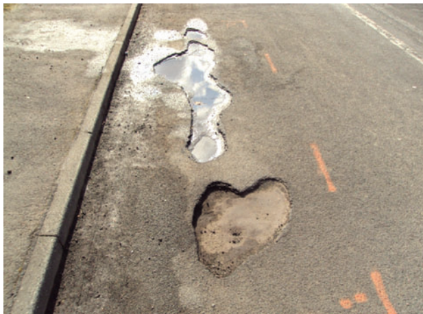
Figure 7.38 Potholes
