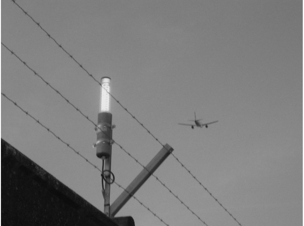
Figure 15-22 Low intensity neon obstacle light, (Photo: M. Mašaš)
