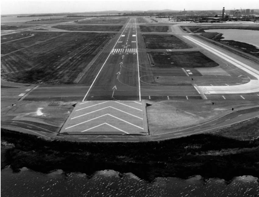
Figure 5-5 EMAS installation at Boston Logan Airport, courtesy ESCO ZODIAC Company (Photo: David J. Heald, C.M.)
