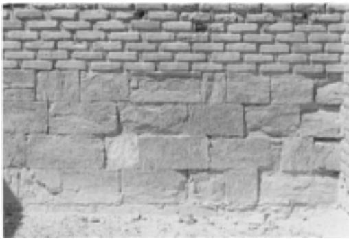
Stone and brick construction, Qasr al-Tuba, Jordan
