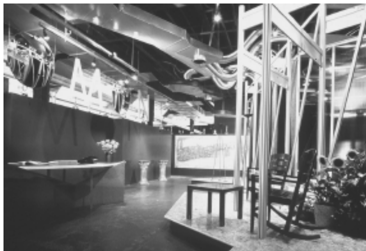
Figure 3.16 An example of multidirectional concentrated distribution.
