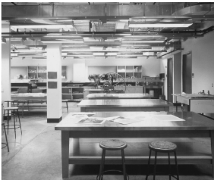
Figure 3.14 An example of direct/indirect distribution.
