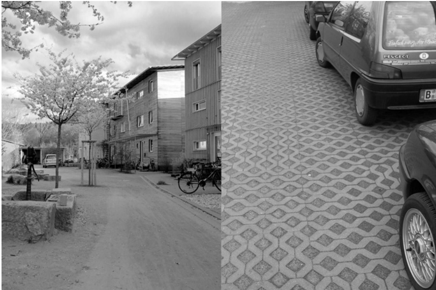
Figure 4.31 Minimise impermeable surfaces
