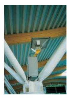
Detail of upward lights at the junction to the columns (photographer Derek Phillips).
