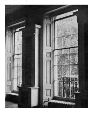
Figure 3.3 A window at the Architectural Association building in London, where the reveals are splayed to balance the contrast of light at the window. The splays are used also to conceal shutters. (Copyright Phillips, Derek, Lighting in Architectural Design, McGraw Hill, 1964, p.40)
