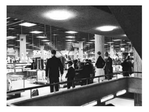
Figure 3.2 An early example of unshielded light sources being used as disability glare sources in a Rotterdam store, to inhibit the views of pipework and ducting above the louvred ceiling. (Copyright International Lighting Review)
