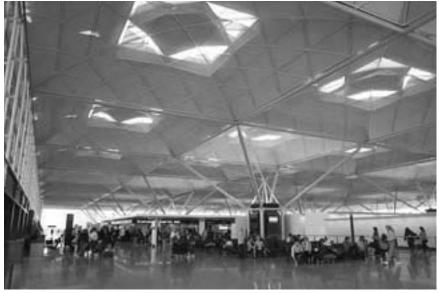
The deep, single-storey building at Stansted Airport allows the whole interior to be flooded with daylight from carefully designed roof lights. (Photographer Derek Phillips)
