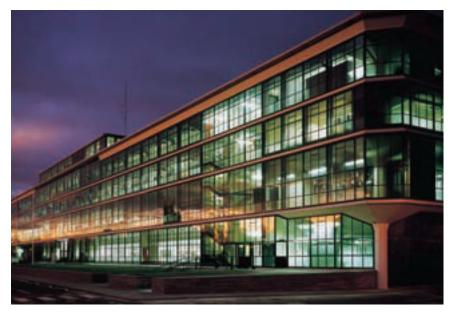
practical type available. The amount of light derived from the method used would have been rather low. The lights are visible at high level in the picture and a more suitable method would have been to have had local sources close to the work.
