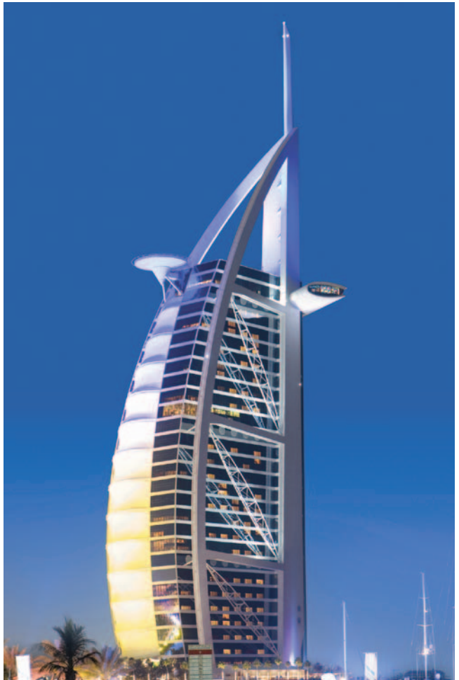
Massive steel supports create Burj al Arab's distinctive sail shape.
