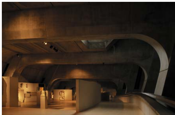
▲ 6.31 Concrete frames extend over the galleries and corridor. The sloping columns express the hill-side embedment of the building.
