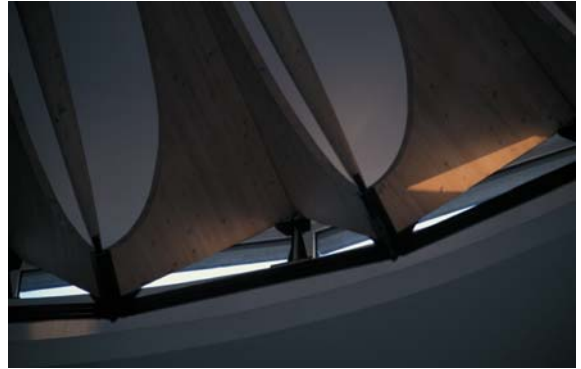
▲ 6.2 Refined timber struts connect to the steel rod tension-ring and the rafters with deepened ends.
