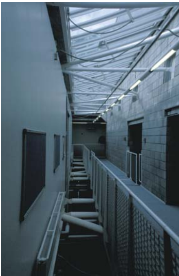
▲ 2.10 Roof and first floor diaphragm bracing.
