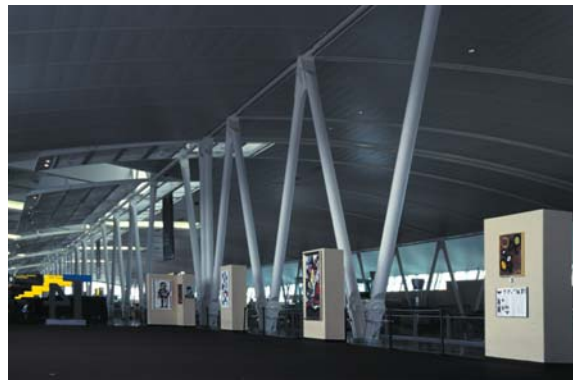
▲ 5.18 V-struts separate ticketing areas to the left from a circulation area and retail outlets on the floor beneath.
