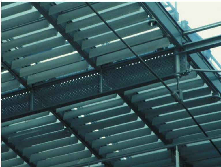
▲ 8.21 Schools of Geography and Engineering, Marne-la-Vallée, Paris, France, Chaix & Morel, 1996. A finely perforated web of a steel beam.
