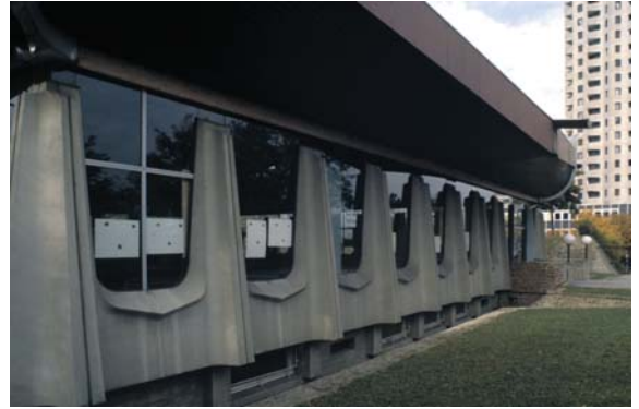
▲ 6.29 The exterior wall is structurally separated from the roof by glazing.
