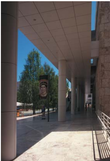
▲ 4.17 A colonnade supporting an elevated walkway alongside an external wall.
