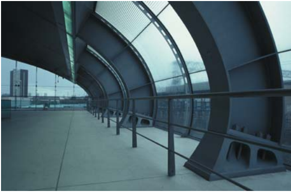
▲ 7.29 Stratford Regional Station, London, England, Wilkinson Eyre, 1999. Curved frames spring from cast-steel bases.
