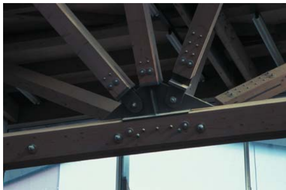
▲ 7.24 Web members connect to a truss bottom-chord.
