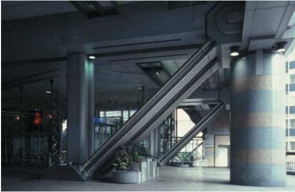
▲ 5.38 125 Alban Gate, London, England, Terry Farrell, 1992. A transfer-truss diagonal member poses a potential danger to passers-by.
