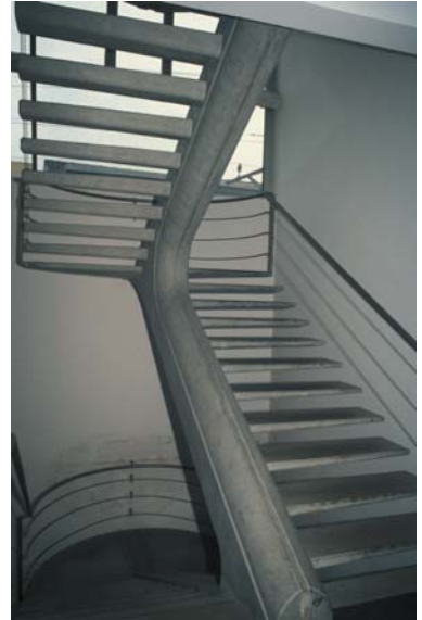
▲ 7.7 Rounded precast concrete stair stringer.
