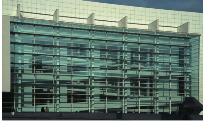
▲ 6.20 Museum of Contemporary Art, Barcelona, Spain, Richard Meier Architects, 1995. Exterior glazed wall to the ramp-hall with the ramp structure behind.
