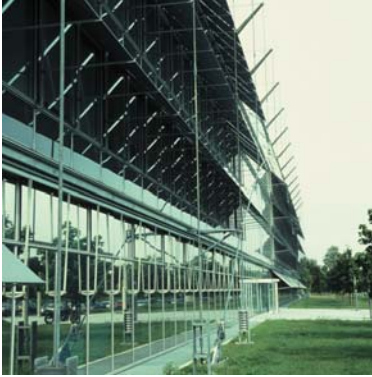
▲ 3.52 Exterior tension rods and springs.
