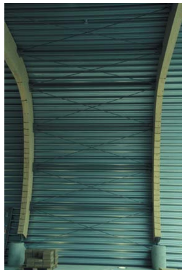
▲ 7.9 Fine diagonal bracing reads as 'stitching'.
