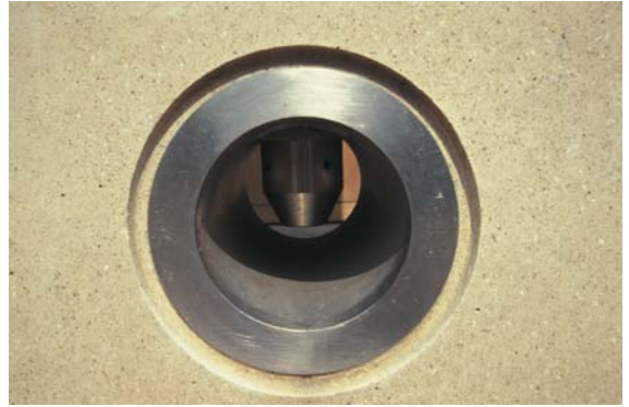
▲ 7.43 A post-tensioning node detail.
