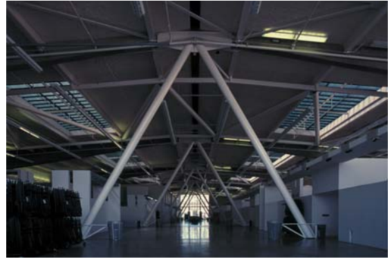
▲ 5.39 California College of the Arts, San Francisco, USA, Tanner Leddy Mantum Stacy, 1999. Light steel frames prevent injuries from the 'Nave' brace members.
