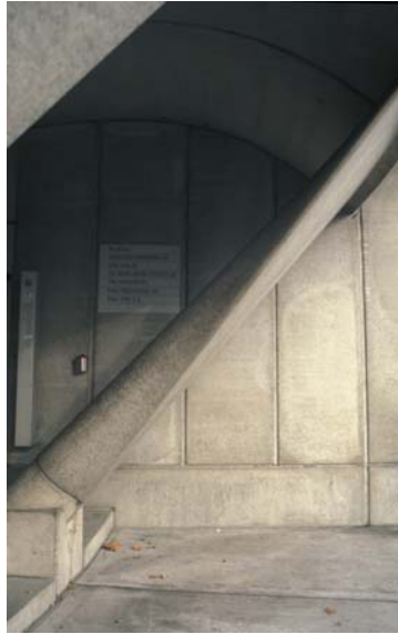
▲ 7.6 Perimeter blade-like pier.
