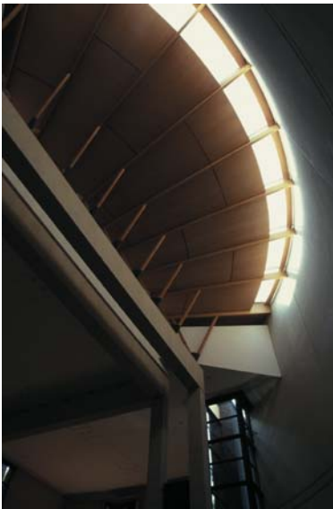
▲ 6.26 The timber roof is propped off an outer frame.
