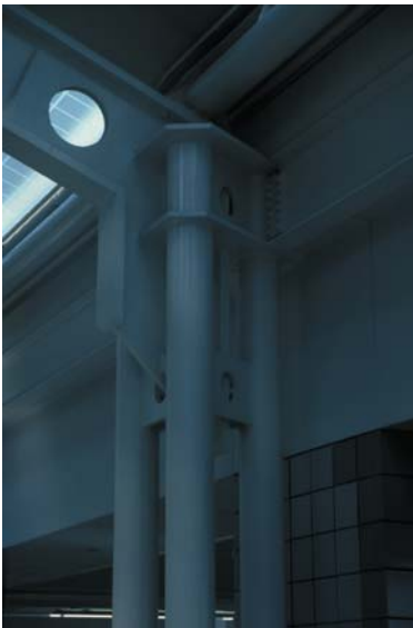
▲ 7.13 Beam-column junction.
