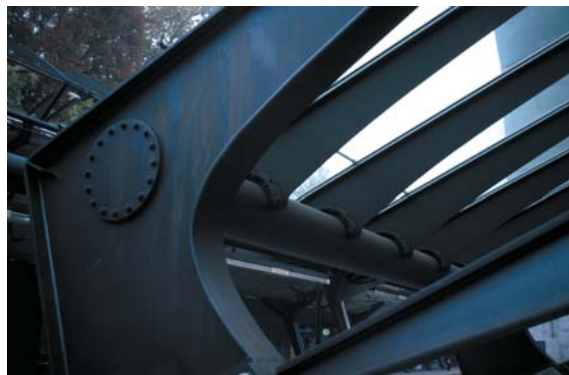
▲ 7.28 Upper cantilever-to-torsion-beam connection, with smaller canopy cantilevers in the background.
