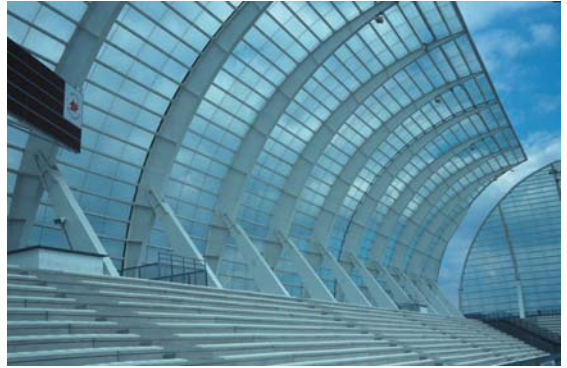
▲ 3.14 Wall ribs, props and longitudinal girts.
